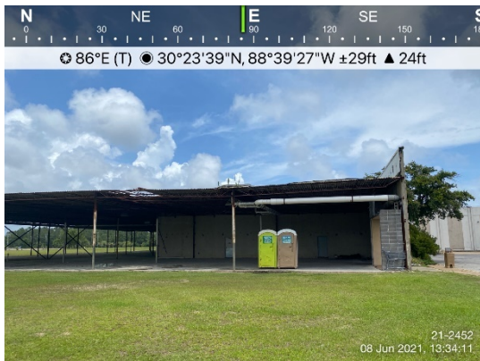
13) View of the subject interior portion that adjoins the Belk Property
