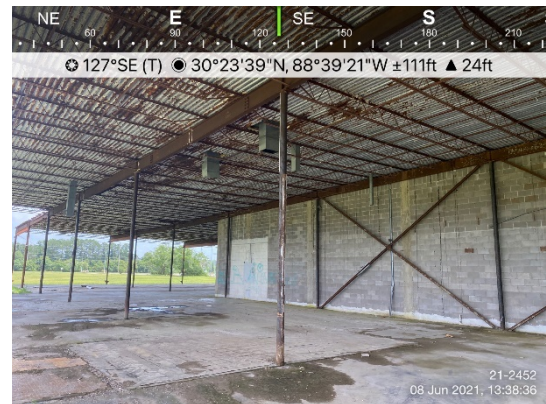
14) View of the subject interior portion that adjoins the Belk Property
