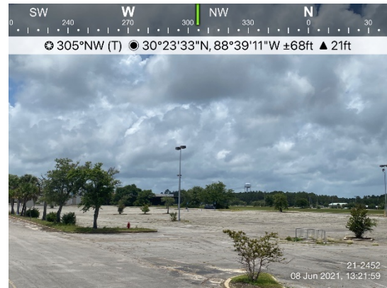
8) View of the subject's paved parking area
