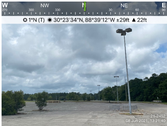
7) View of the subject's paved parking area
