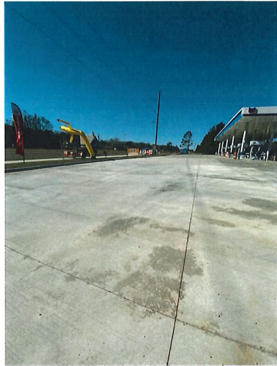
Looking west in front of Store
