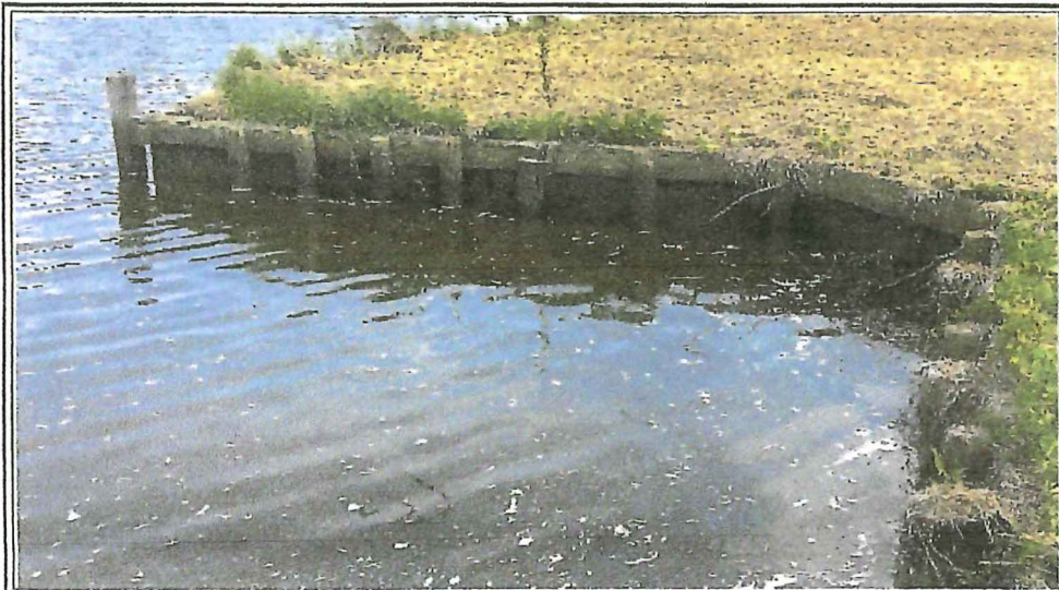
ADDITIONAL BOAT SLIP
