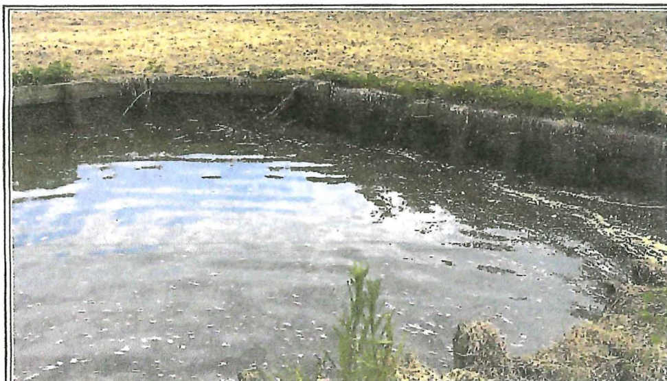
ADDITIONAL BOAT SLIP
