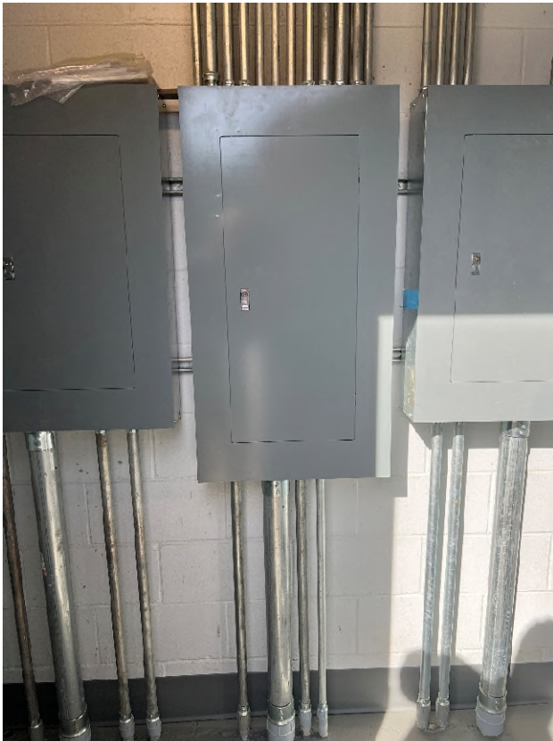
Fig 1. Install electrical panel tags on panel covers
