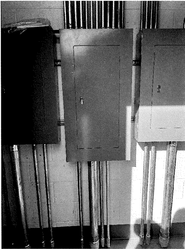
Fig 1. Install electrical panel tags on panel covers
